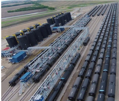
Altex Lashburn Crude Terminal
